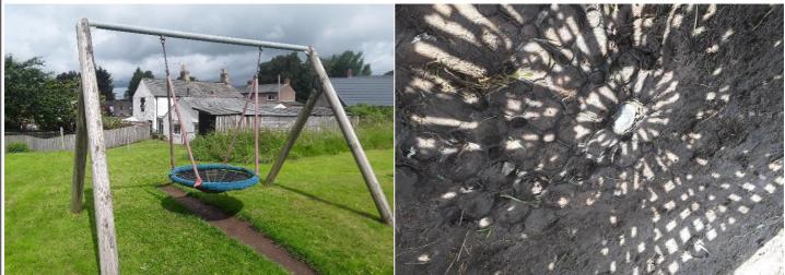
Finding: Fixing Pins have been installed in the impact area Action: Remove pins from impact area
