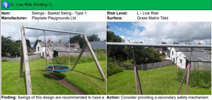
**Finding:** Swings of this design are recommended to have a **Action:** Consider providing a secondary safety mechanism secondary safety mechanism fitted to prevent collapse of the seat
