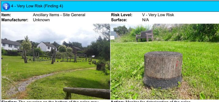
**Finding:** The covering on the bottom of the poles may cause rot, due to been damp. N.B Stimmer damage can also lead to rot
